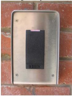
When you swipe a card across the front of the reader, the light will flash green to indicate that the reader has read the card. This is shown in the picture below.
